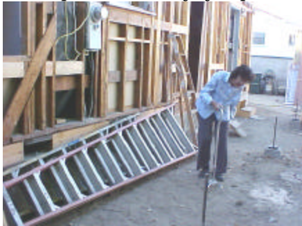
Aug. '03: looking at the construction
